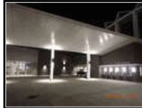
Front of building
