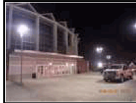
Front of building
