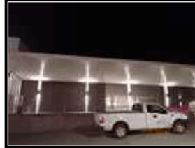
Front of building
